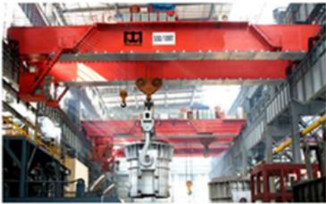
Foundry Industry Cranes
