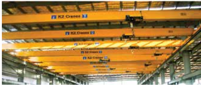
105+ Cranes in one Roof
