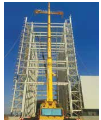
Installation at 45 Mtr Height
