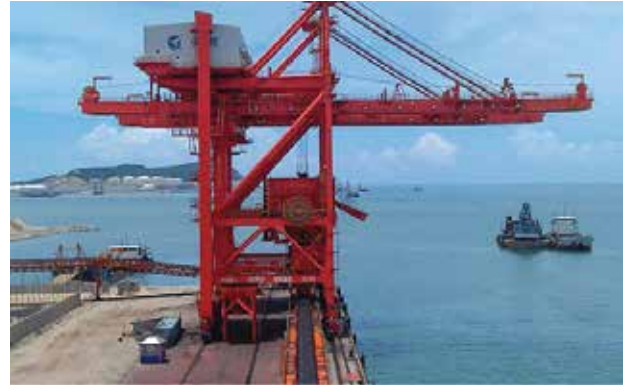
Ship-to-Shore Gantry Cranes
